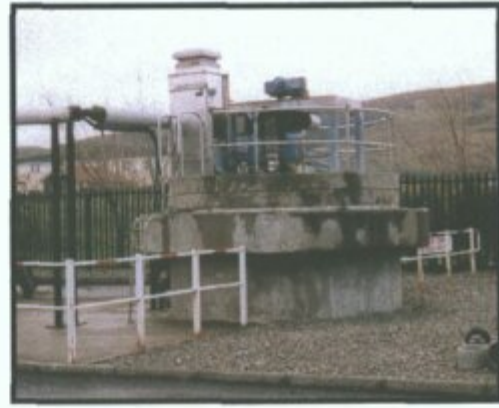
PLATE 3.3.2 MONOMUNCHER & PICKET FENCE THICKENERS
