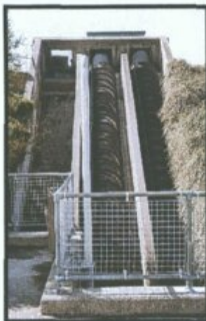
PLATE 3.2.1 SCREW PUMPS, FINE SCREENS & GRIT CHAMBER
