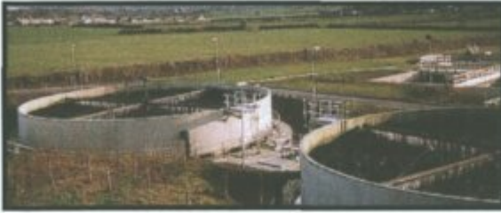
PLATE 3.6.1 TRICKLING FILTER, DISSOLVED AIR AERATION TANK & TIDAL TANK
