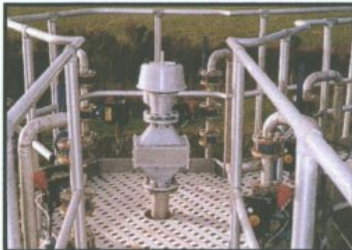
PLATE 3.6.5 VACUUM AND RELEASE VALVE, GAS MIXING PIPES & GAS HOLDERS
