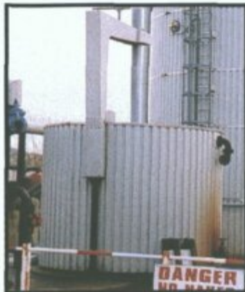
PLATE 3.3.5 GAS HOLDER & GAS COMPRESSOR FOR MIXING
