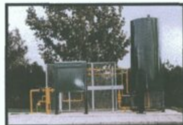
PLATE 3.2.6 THE GAS HOLDER, CHP UNIT & FLARE STACK
