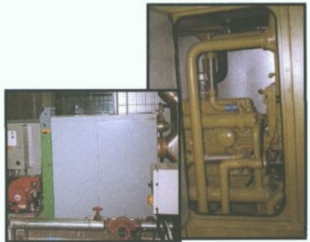
PLATE 3.4.4 THE HEAT EXCHANGER, BOILER AND CHP UNIT
