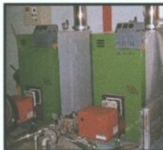
PLATE 3.6.4 HEAT EXCHANGER UNIT, BOILERS & CHP UNIT
