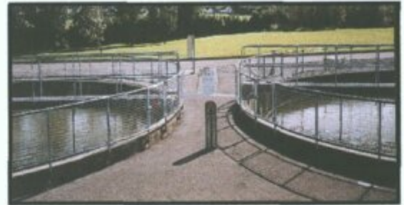
PLATE 3.2.3 THE AERATION TANK & THE TWO SECONDARY CLARIFIERS
