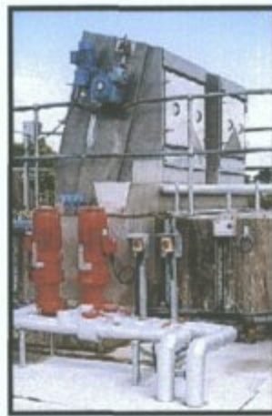
PLATE 3.2.1 SCREW PUMPS, FINE SCREENS & GRIT CHAMBER
