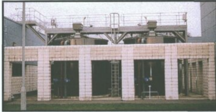
PLATE 3.4.2 THE TWO PICKET FENCE THICKENERS
