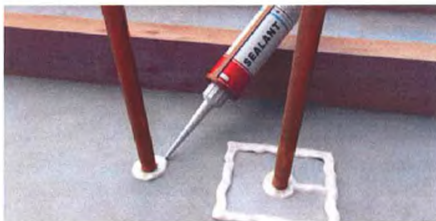
Figure 18 Sealant Placed Around Pipes to Achieve Good Air Tightness source google.ie
