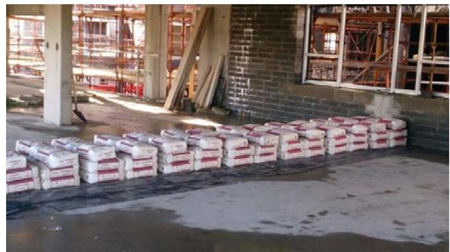
Figure 8. Load test on first floor slab
