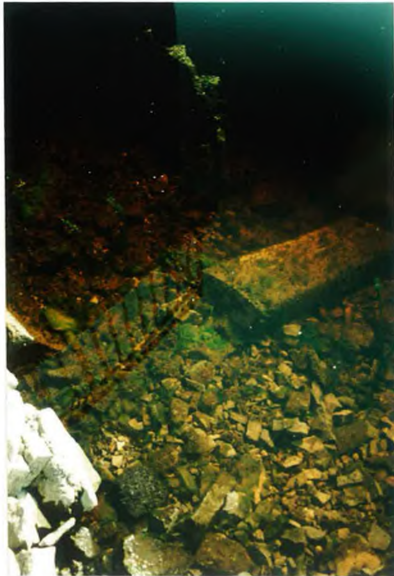
Plate 2: Brown and green gelatinous materials found in the littoral zone of Lough Gill. Plate shows submerged concrete structure with attached growth. Plate from the water pump house in Tobernalt Bay on the 2 nd June 1998.
