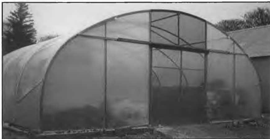
Plate. Polyethylene tunnel at Barroe House Farmyard
