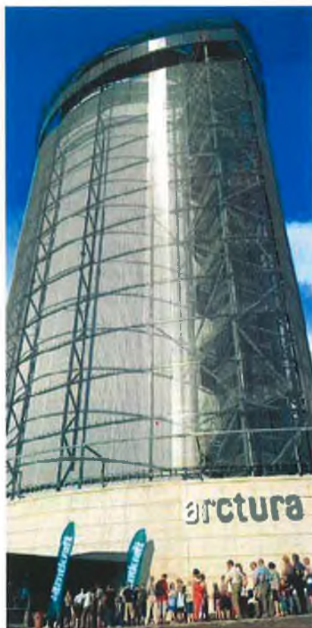
Figure 19 A 65m high accumulator tank at Ostersond, Sweden with a restaurant on the top floor.
