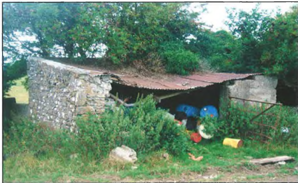
Figure 6.11. The Dispatch Centre as it Stands Today
