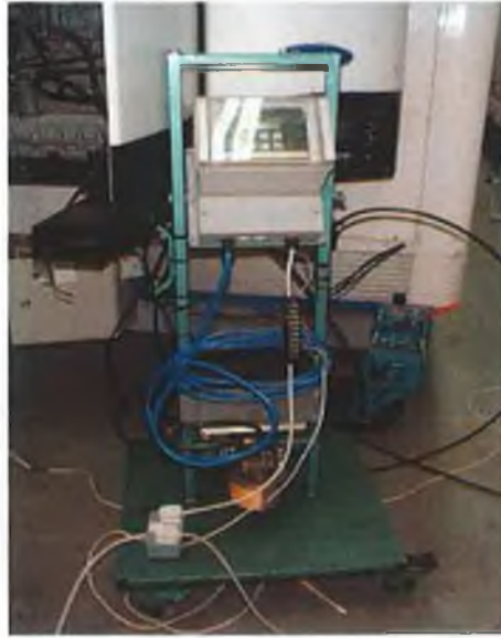
Figure 3A Flow Meter
