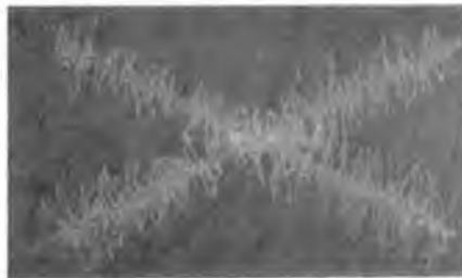
Figure 3.5 Filiform corrosion photograph
