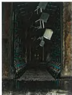
Treatment spray tunnel
