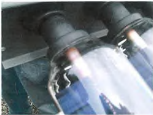
Figure 28: Copper tubing of Evacuated tube (ET)
