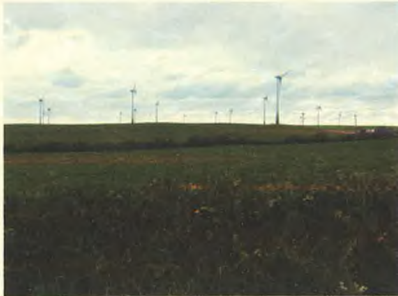
Figure 50: Ballywater, Co. Wexford
