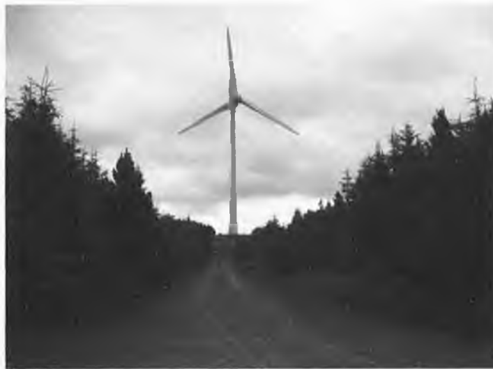
Figure 5: Case Study Turbine
