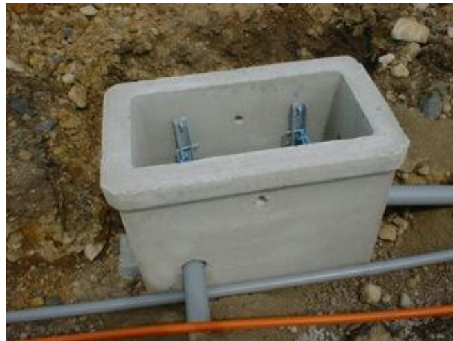
Figure 2: Typical precast underground service chamber box
