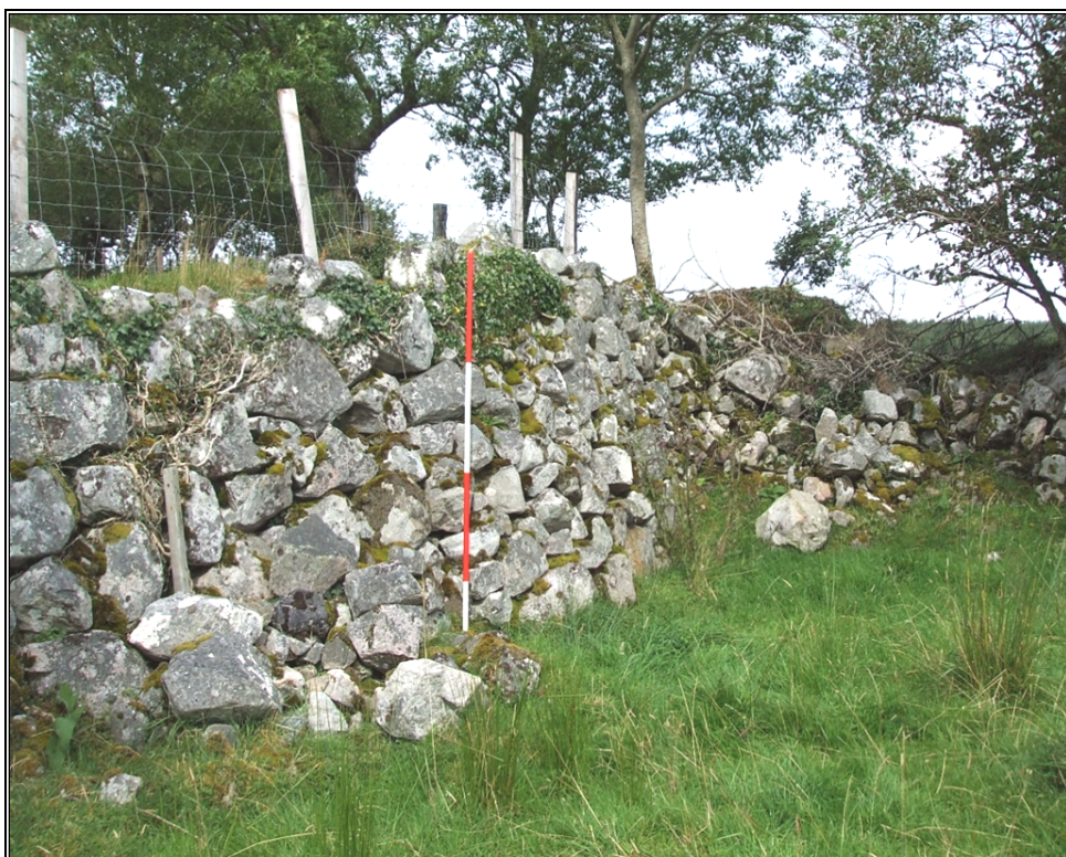
Plate 6.1 Ballydawley revetment south face
