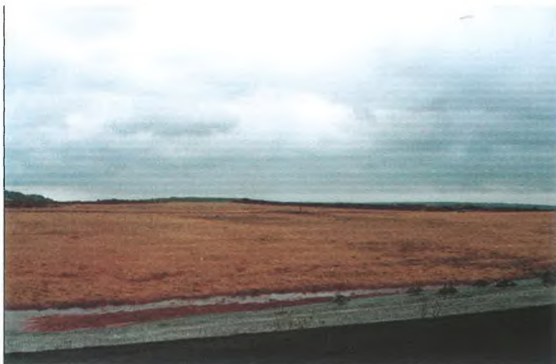
Plate 1.2. View of section of mud stack shortly after application of straw thatch to suppress dust.
