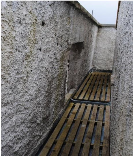
On the Roof
